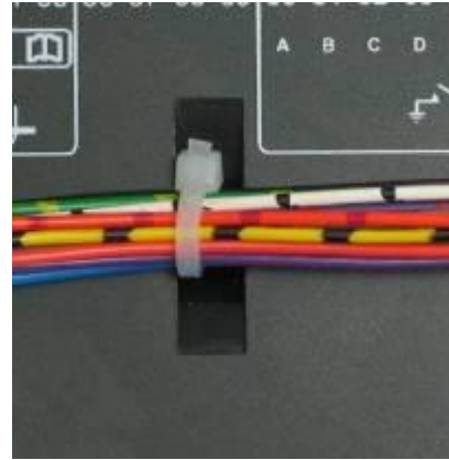
With Cable And Tie In Place
